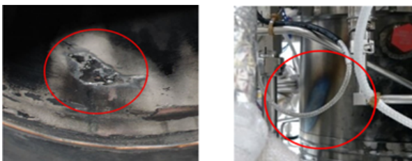
Fig. 9 Damages to inner wall(left) and outer wall(right) of upper stage engine 6G combustion chamber during the combustion test.
