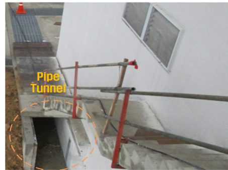
Fig. 10 Pipe tunnel.
