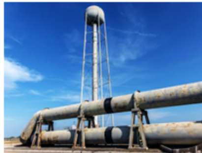
Fig. 14 High water storage tank support structure.
